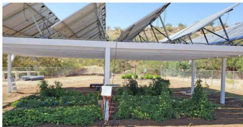
An experimental agriphotovoltaic setup at the University of Arizona, KILLAMATOR (CC BY-SA)
