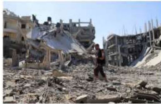
Dire straits: An injured man walks among the rubble of his house to inspect the damage in Sabra in Gaza City on Wednesday. REUTERS
